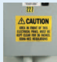
Hazard warning signs
